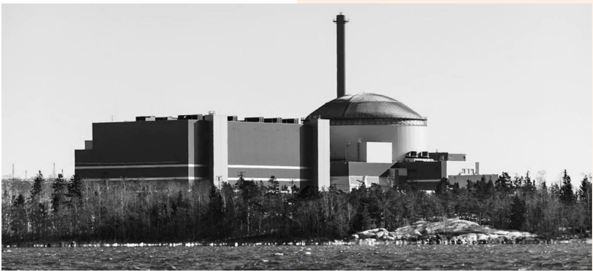
Olkiluoto 3 i Finland.
